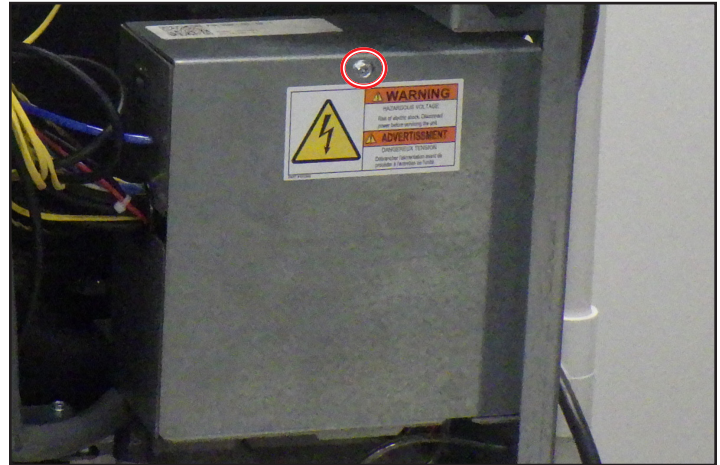
Fig. 1. Electrical box cover screw location.
