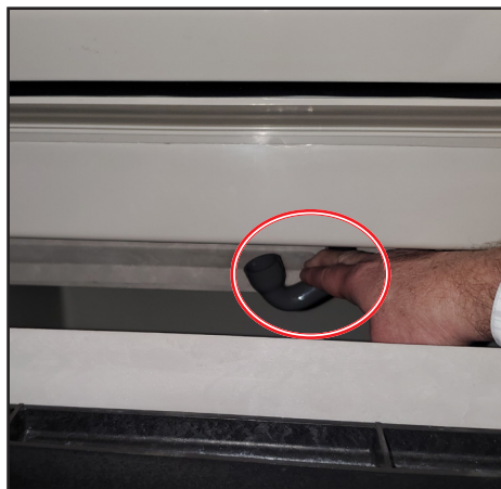
Fig. 1. Disconnect the drain hose from the sump.
