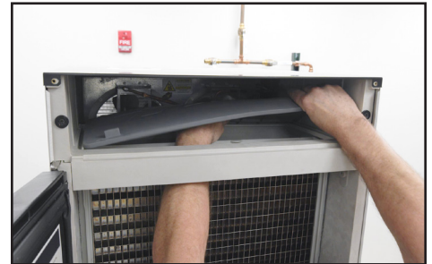
Fig. 7. Remove the evaporator cover.
