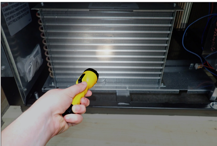
Fig. 3. Use a flashlight to inspect and confirm that the coil is clean.
