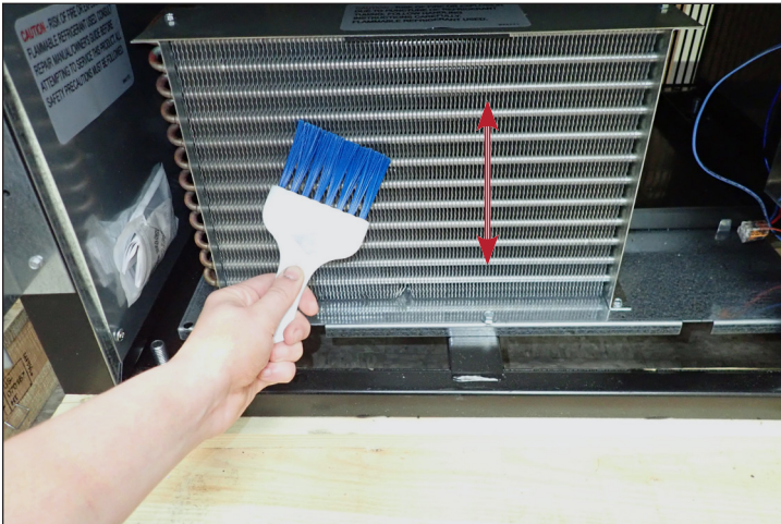
Fig. 2. Never brush across the coil fins.
