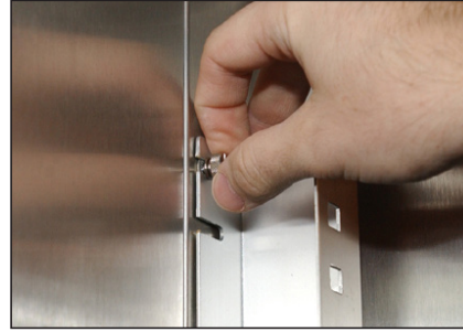
Fig. 1. Pilaster installation on cabinet sidewall.
