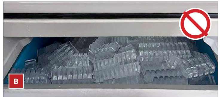
Fig. 10. Ice bins with (A) and without (B) a drop-zone deflector.
