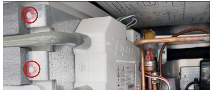
Fig. 2. TrueZone UV system side view. TrueZone bracket screw locations.
