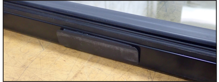
Fig. 17. Wire cover located in the hinge-side of the door in the center.
