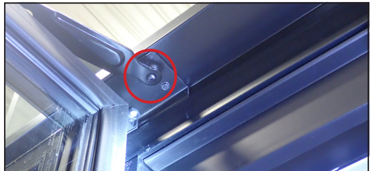
Fig. 15. Hold open bracket screw location at the top of the door.
