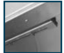
Stainless steel thermal breaker (interior)
