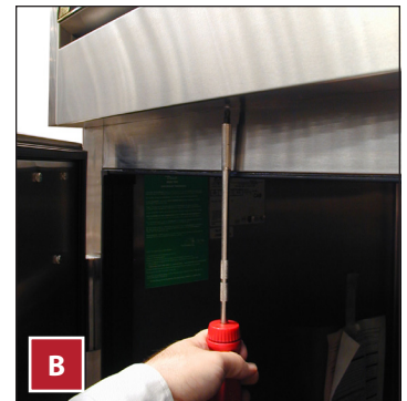
Fig. 2. If accessible, clean the condenser coil. Never brush across coil fins.
