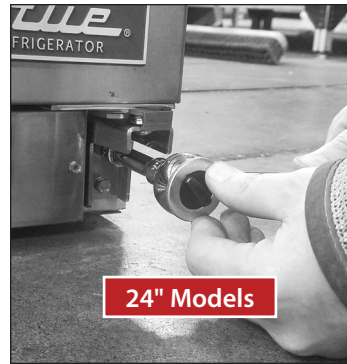
Fig. 1. The 24 and 27 models use different lower hinges.
