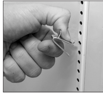
Fig. 1. Installing top tab of shelf clip.
