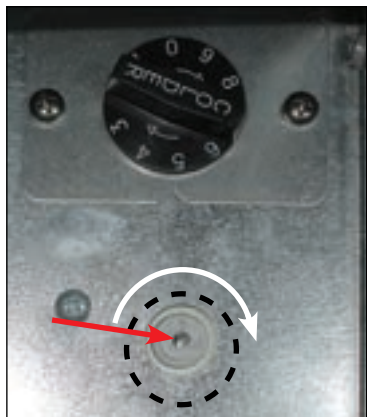
Rys. 2. Turn the actuating gear clockwise until the contacts click.
