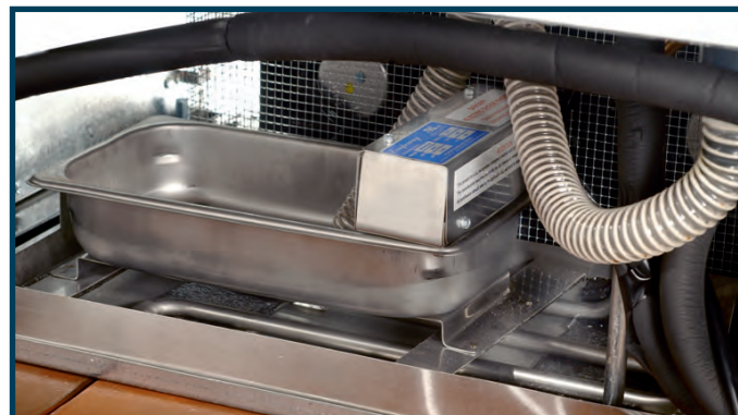
Condensate Heater Pan/Bracket Kit (pictured without back screen).
