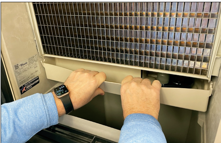
Fig. 4. Pull the sump tank forward and push down.
