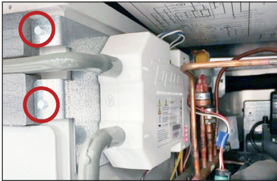
Fig. 3. TRUEZONE UV system side view. TRUEZONE bracket screw locations.
