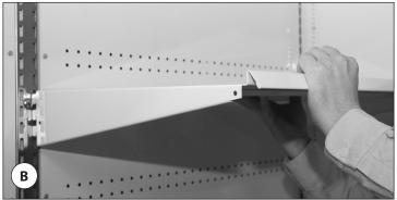
Fig. 2. Hook the shelf supports into the shelf standards.
