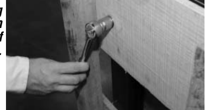
Removing skid from bottom of cabinet.
